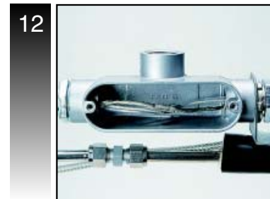
Insert remaining heating cable through second connector union and tighten securely.
