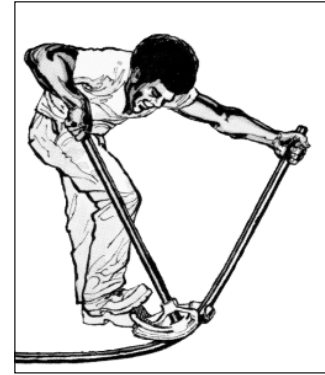
Workperson using a thin wall conduit bender with Temptube.
